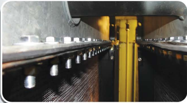
All damaged and worn components are replaced.
